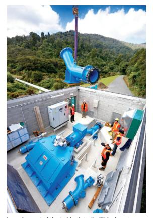
Lowering part of the turbine into the Wainuiomata hydro-electric generator building
