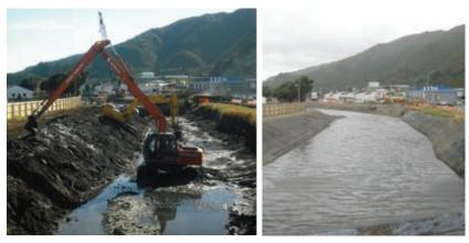
Diggers removing contaminated sediment from a section of the Waiwhetu Stream upstream of the Hutt Park bridge (left) and the same section of stream flowing naturally again and ready to be planted with native vegetation (right).
