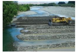
A bulldozer realigning a section of the Waingawa River channel to reduce erosion that is occurring along the left bank.
