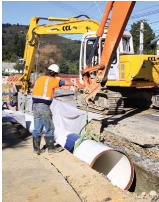
Diggers lift a new section of the Wainuiomata water main into place
