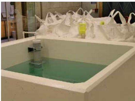
Generating chlorine from saltwater at Te Marua will save an estimated \$80,000 annually. This picture shows the hypochlorite plant's brine tank
