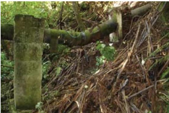
We replaced a vulnerable section of the water main to Karori, across the Kaiwharawhara Stream (pictured), with a new section of pipe buried beneath the streambed
