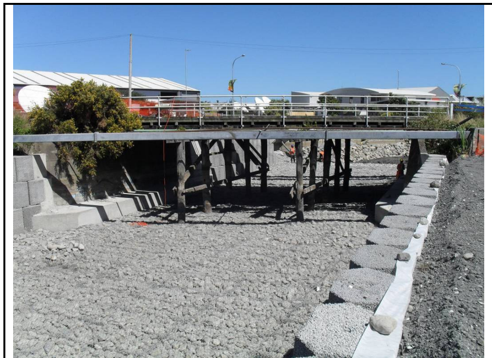
Photograph 8: Looking downstream towards Hutt Park Bridge, following excavation and installation of erosion and scour protection.
