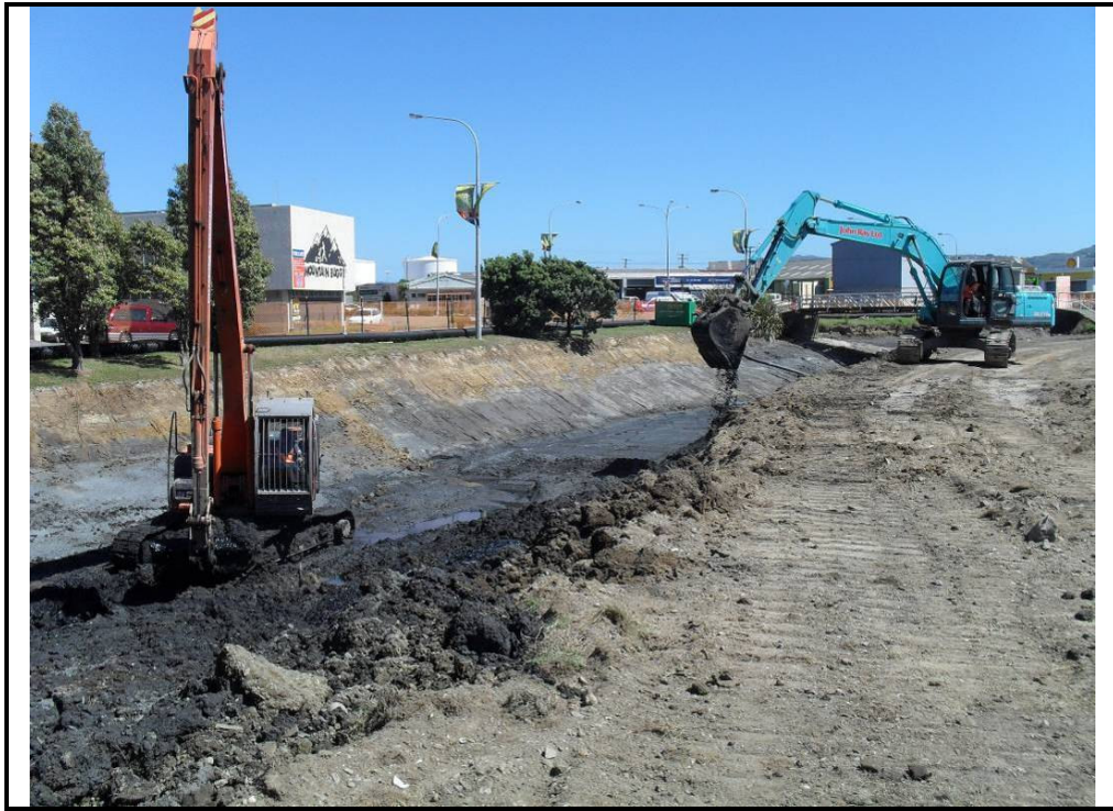
Photograph 3: View looking downstream towards the Hutt Park footbridge that was dismantled during excavation works in this cell.
