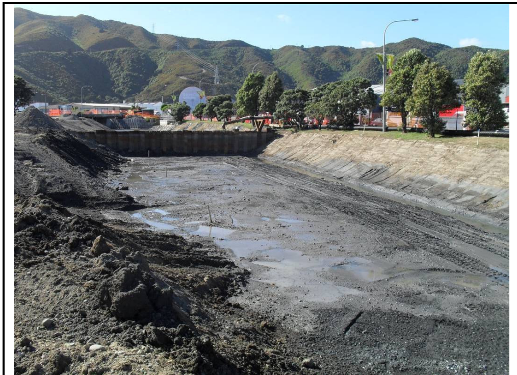
Photograph 5: View looking upstream towards coffer dam 6 following the removal of the contaminated material.
