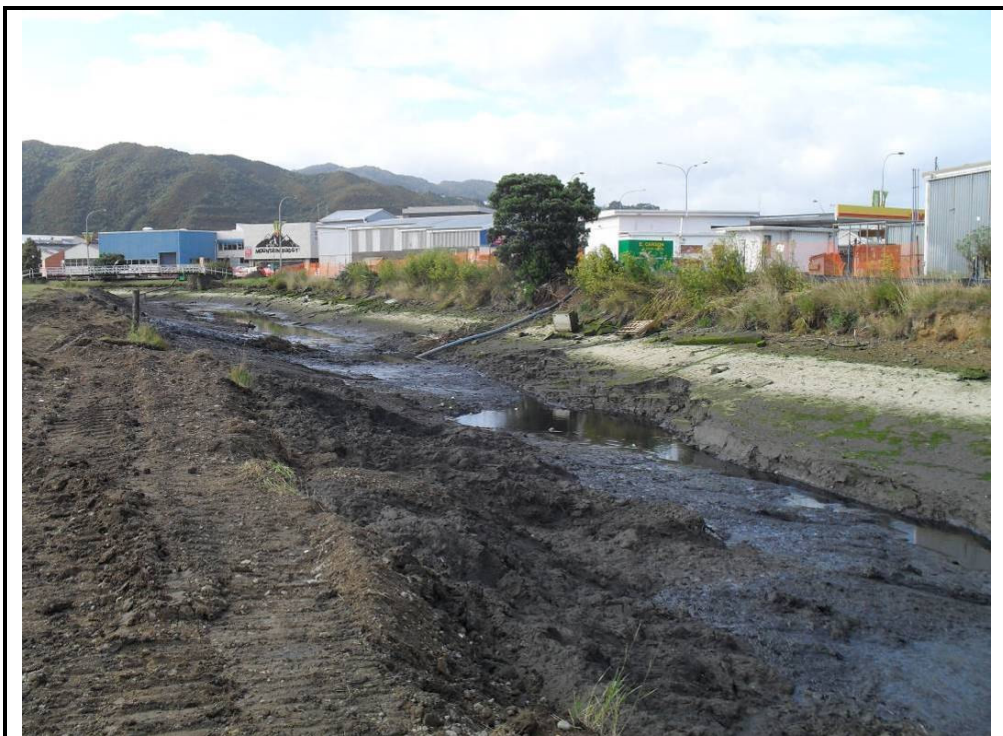
Photograph 2: View looking upstream towards the Hutt Park footbridge that was dismantled during excavation works in this cell.
