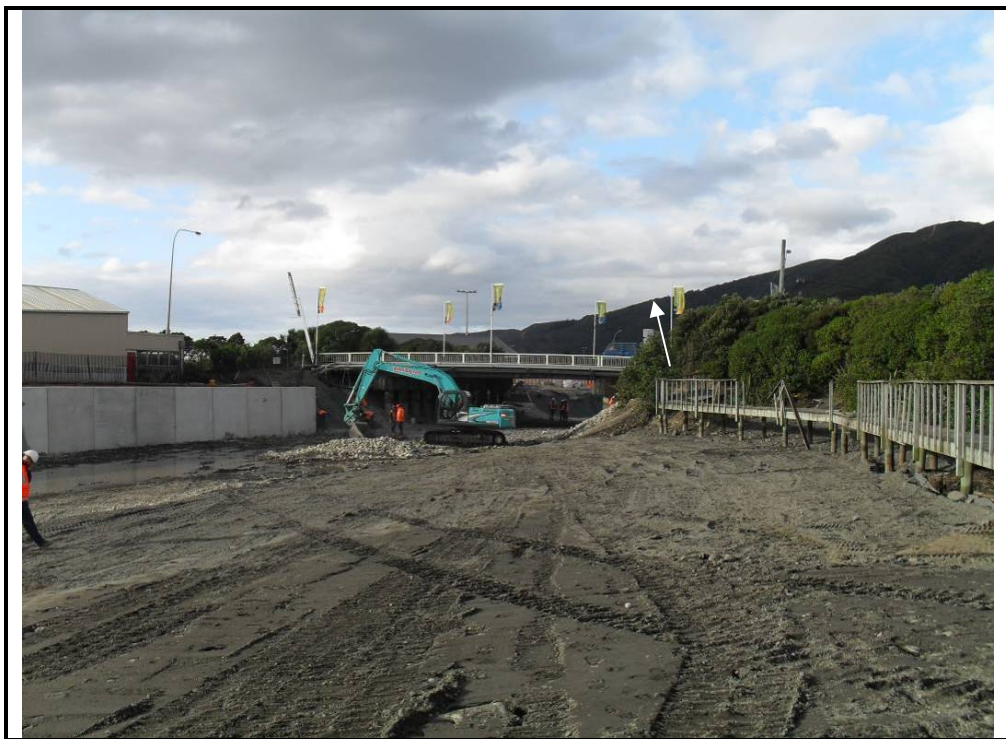
Photograph 10: View looking upstream towards Seaview Road Bridge following the removal of contaminated material, and the rebuilding of the salt marsh.
