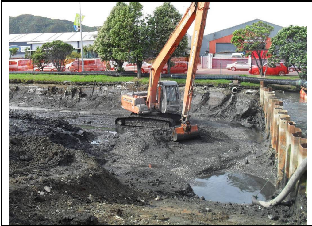
Photograph 3: Cell E at coffer dam 5 during excavation.
