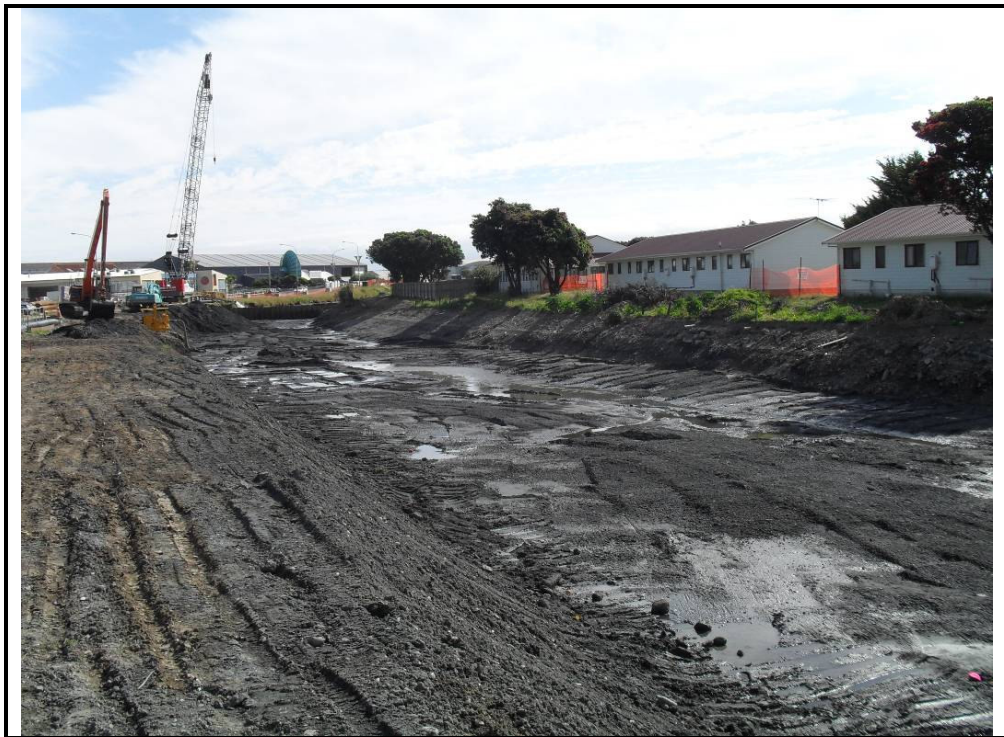
Photograph 6: Cell C/D following excavation.
