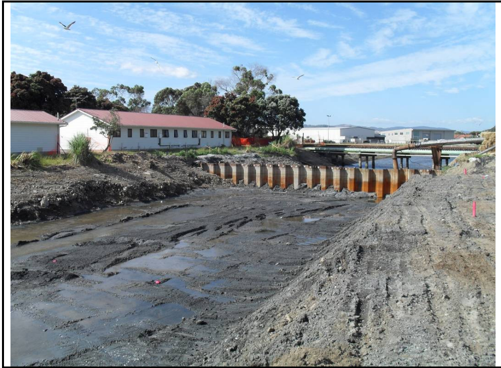
Photograph 3: Looking upstream towards coffer dam 2 following excavation.
