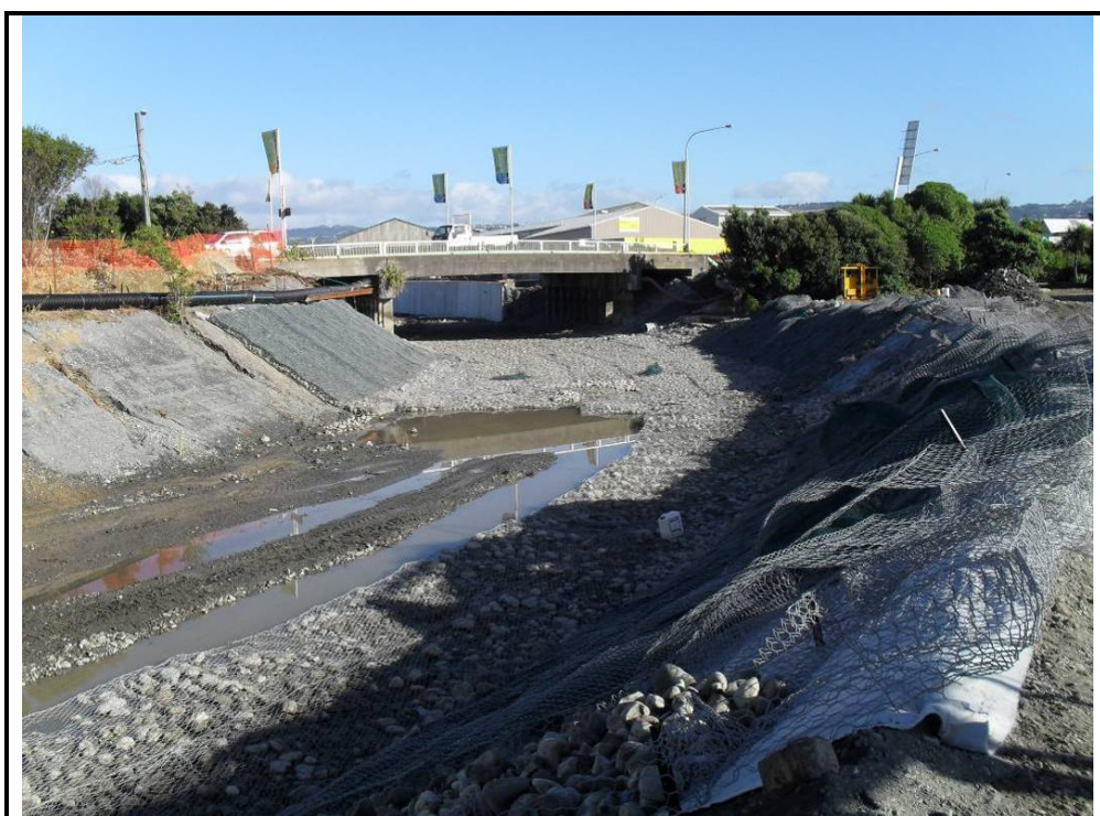
Photograph 4: Cell H looking downstream towards Seaview Road Bridge, following the removal of contaminated material and during the installation of reno mattresses.
