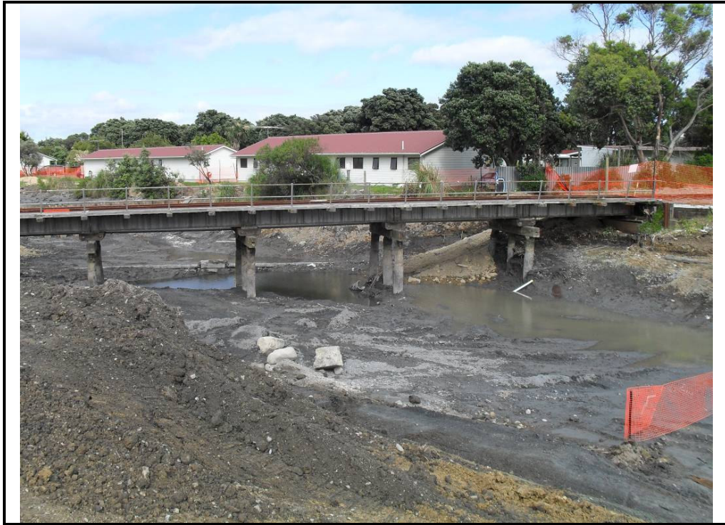
Photograph 5: Looking downstream towards the rail bridge. The gas main can be seen immediately downstream of the bridge.
