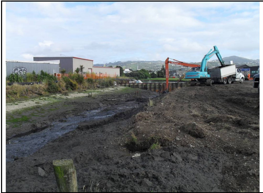
Photograph 1: View looking downstream towards coffer dam 7 during the removal of contaminated material.
