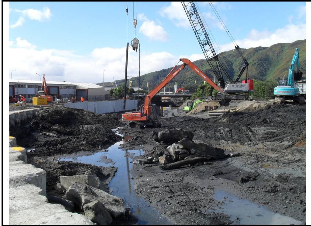
Photograph 3: Cell M looking upstream during the removal of contaminated material
