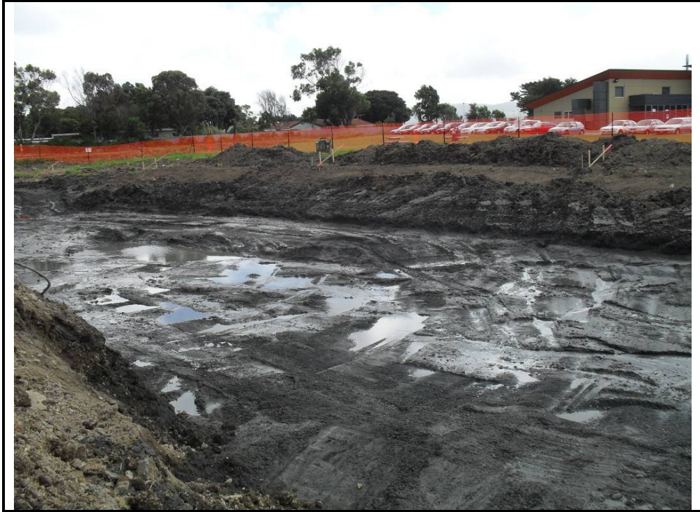
Photograph 3: The stream bed following the excavation of the contaminated material.
