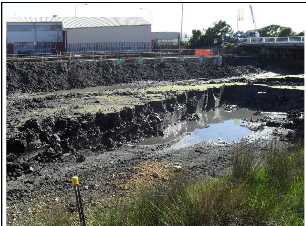
Photograph 5: View looking upstream towards Seaview Road Bridge of the salt marsh in Cell H during the removal of contaminated material.
