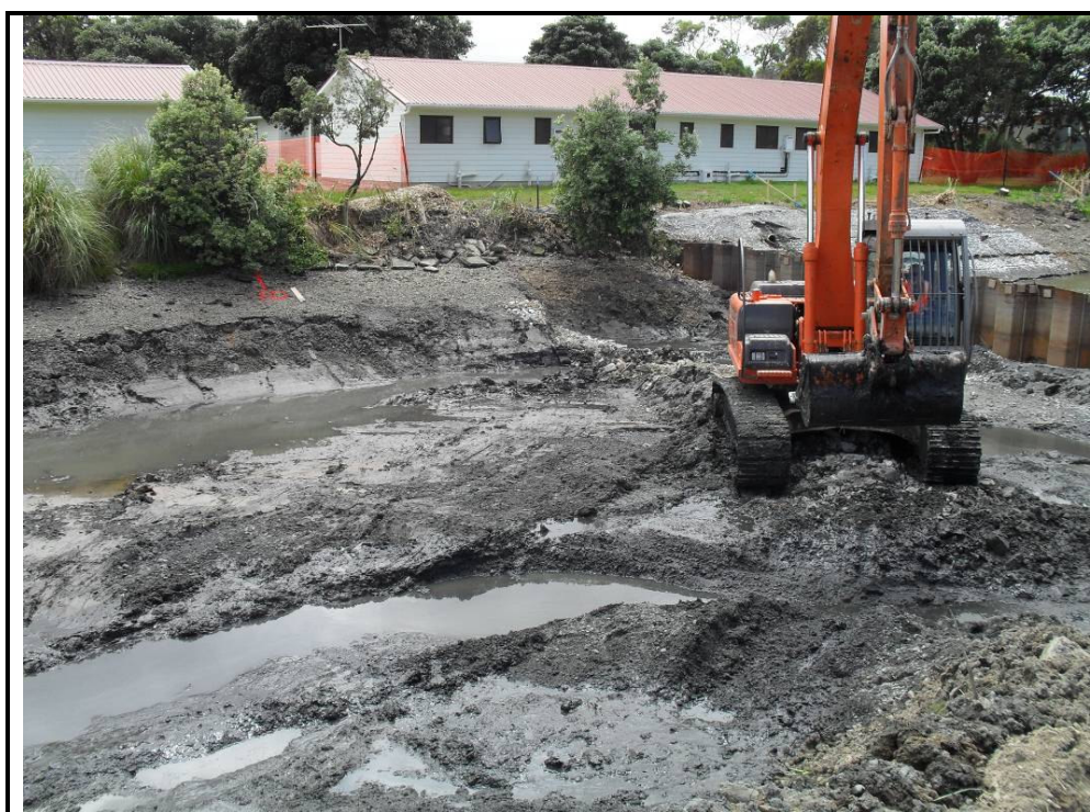
Photograph 2: Cell C during the early stages of excavation. A long-reach excavator was used for Cell C/D and all downstream cells.
