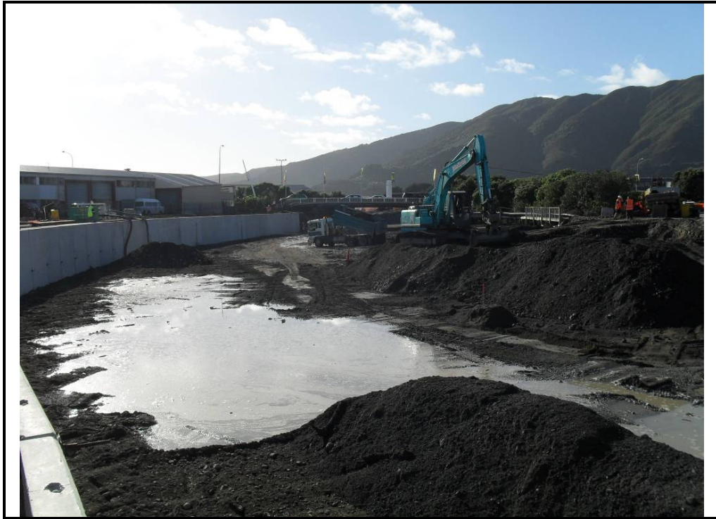
Photograph 5: Cell M looking upstream following the removal of contaminated material and during the re-building of the stream bed level.
