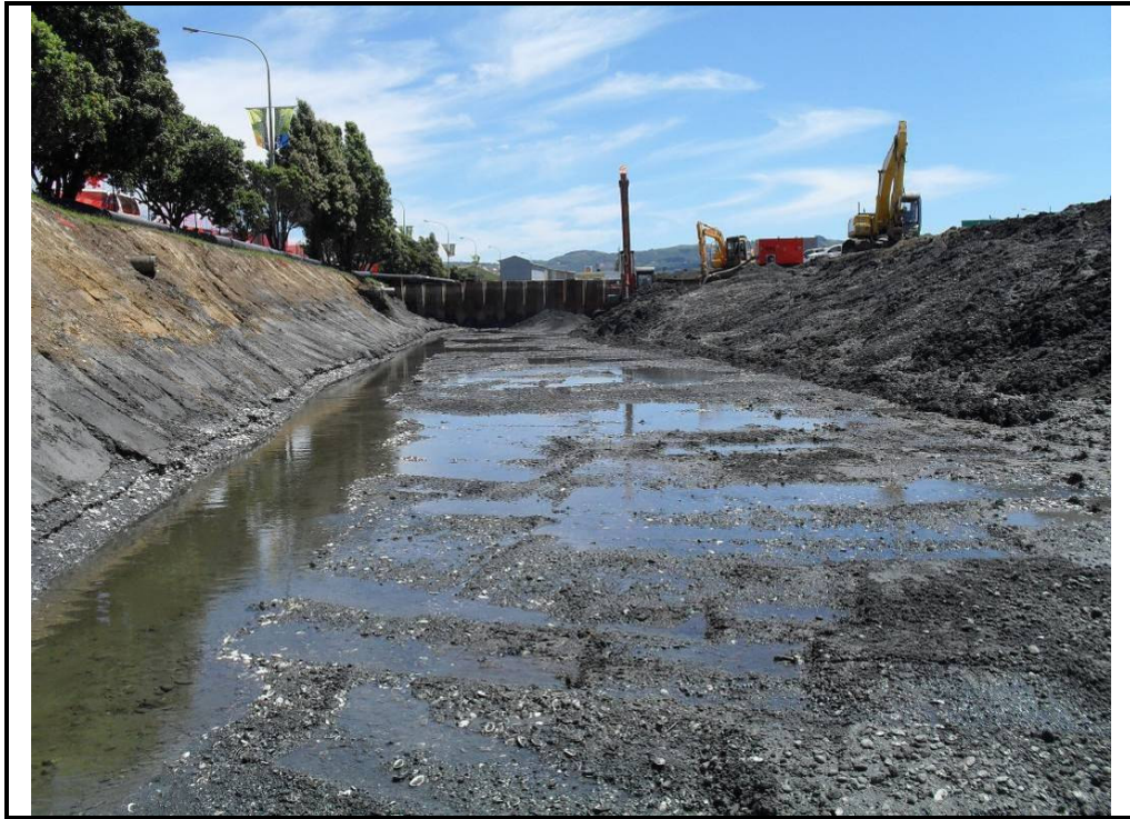
Photograph 5: Looking downstream towards coffer dam 5 following excavation.
