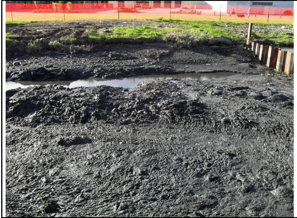
Photograph 1: Cell B immediately downstream of Cofferd Dam 1 prior to the commencement of excavation.
