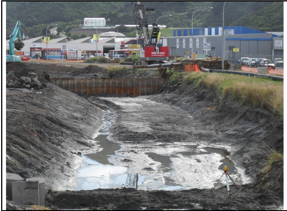
Photograph 1: Looking upstream towards coffer dam 4. Photograph taken from Hutt Park Bridge.
