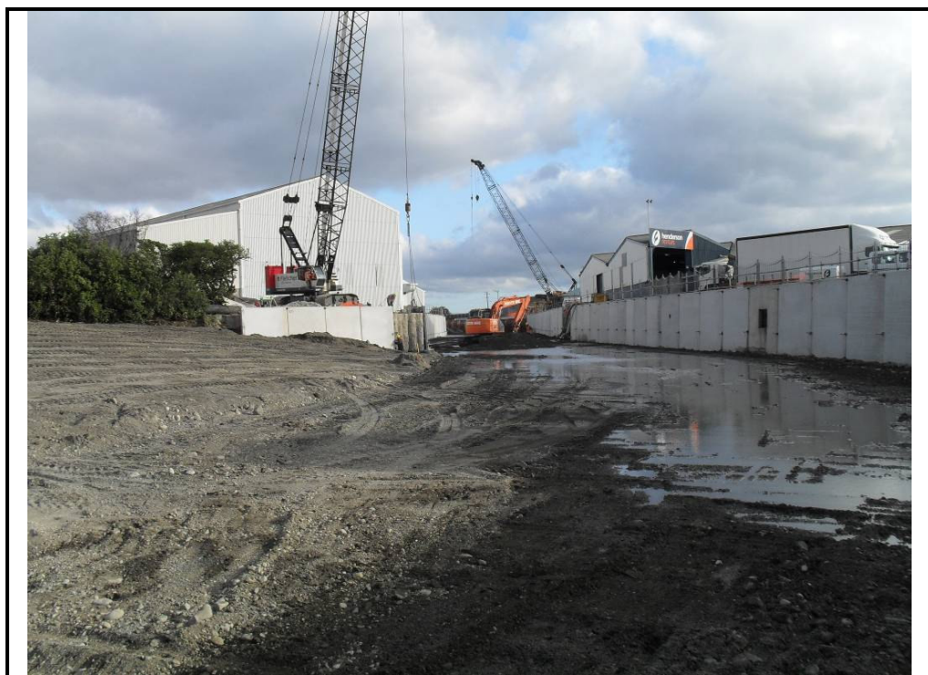
Photograph 6: Cell M (U-channel) looking downstream towards coffer dam 9 following the rebuilding of the salt marsh and the stream bed.
