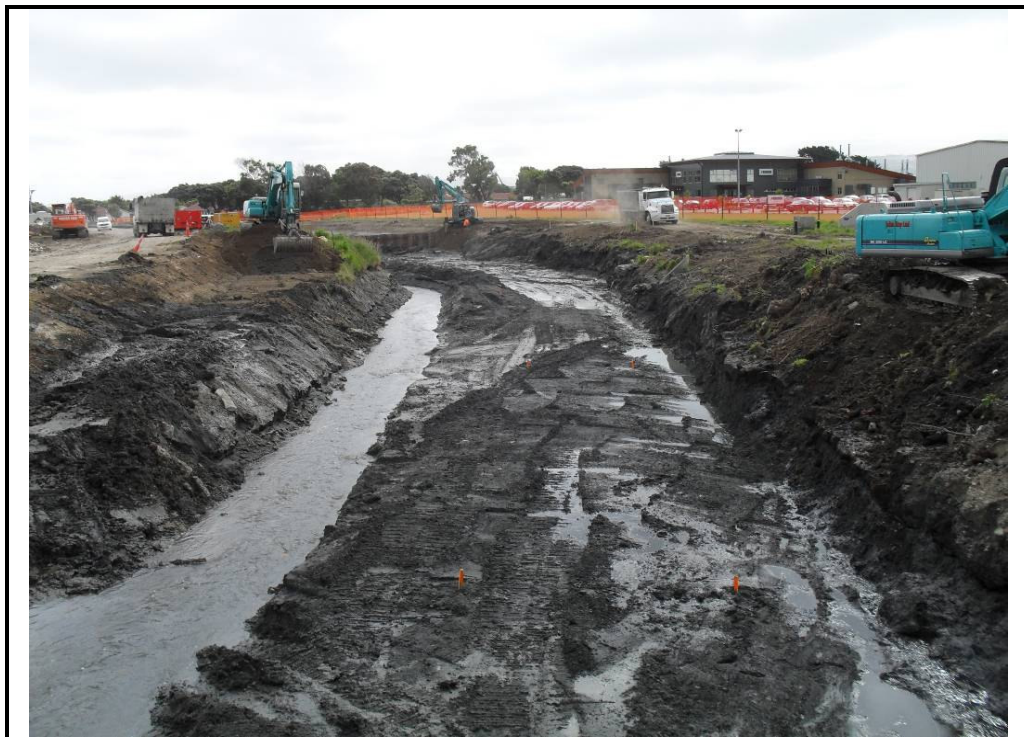
Photograph 4: Cell A looking downstream post-excavation. Orange pegs denote validation sample locations.
