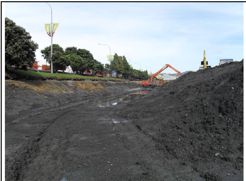
Photograph 2: Cell E during excavation, looking downstream towards coffer dam 5.
