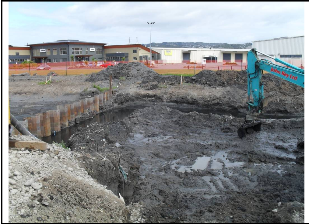
Photograph 1: Excavation works in Cell A. Note diversion channel.
