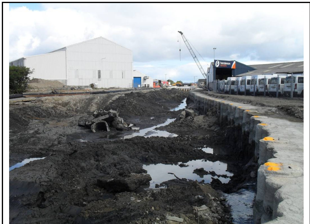
Photograph 2: Cell M (U-channel) looking downstream towards coffer dam 9 prior to the removal of contaminated material.
