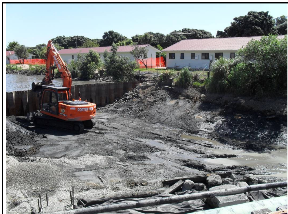
Photograph 6: Looking downstream towards Cofferdam 2. Photograph taken from on top of the rail bridge, the gas main can be seen in the foreground.
