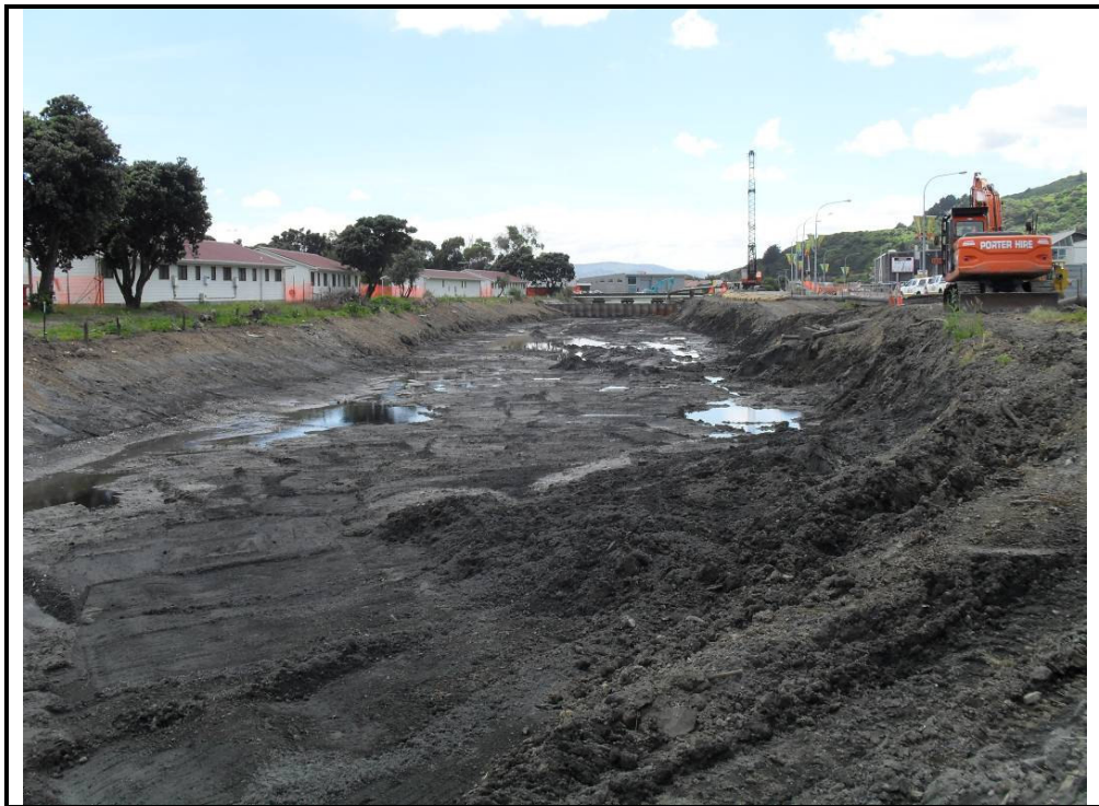
Photograph 4: Looking upstream towards coffer dam 2 following excavation.
