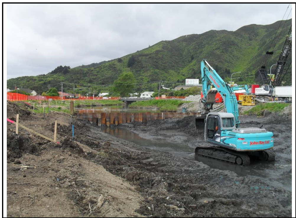
Photograph 2: Looking upstream towards Cofferd Dam 1 during excavation.
