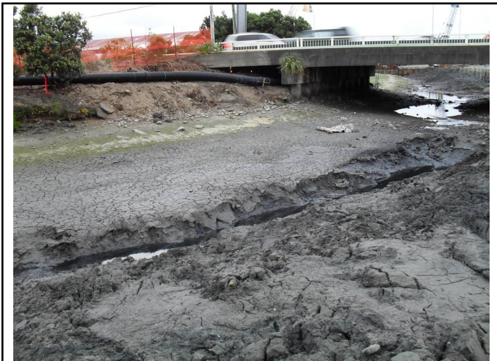
Photograph 2: Cell H looking downstream towards Seaview Road Bridge, prior to the removal of contaminated material.
