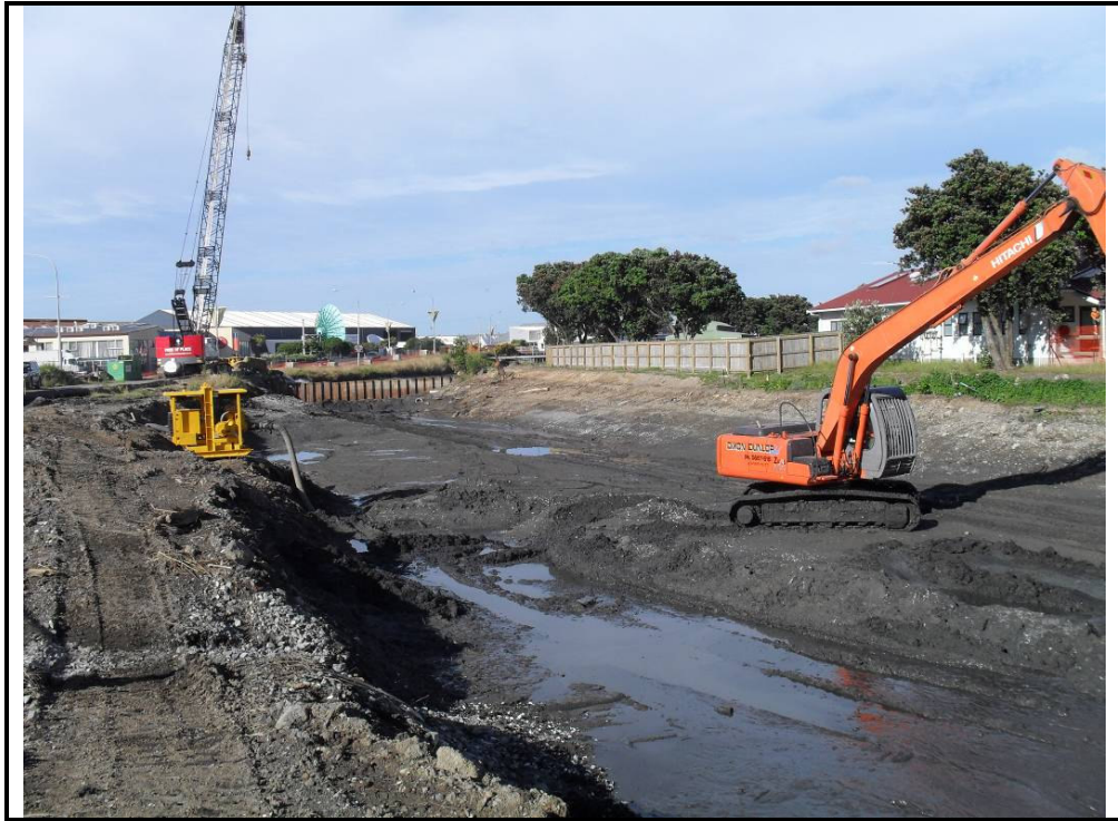
Photograph 5: Cell D during excavation.
