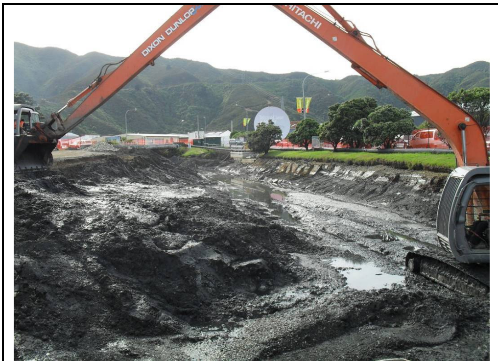
Photograph 4: Looking upstream during excavation.
