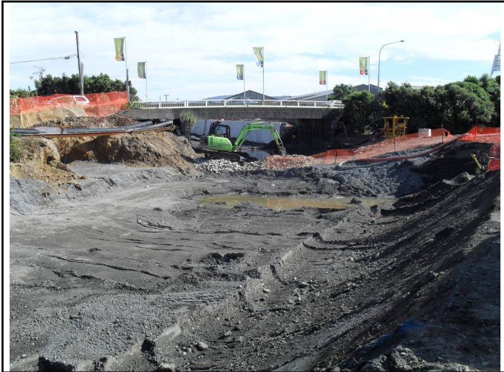
Photograph 3: Cell H looking downstream towards Seaview Road Bridge, following the removal of contaminated material.
