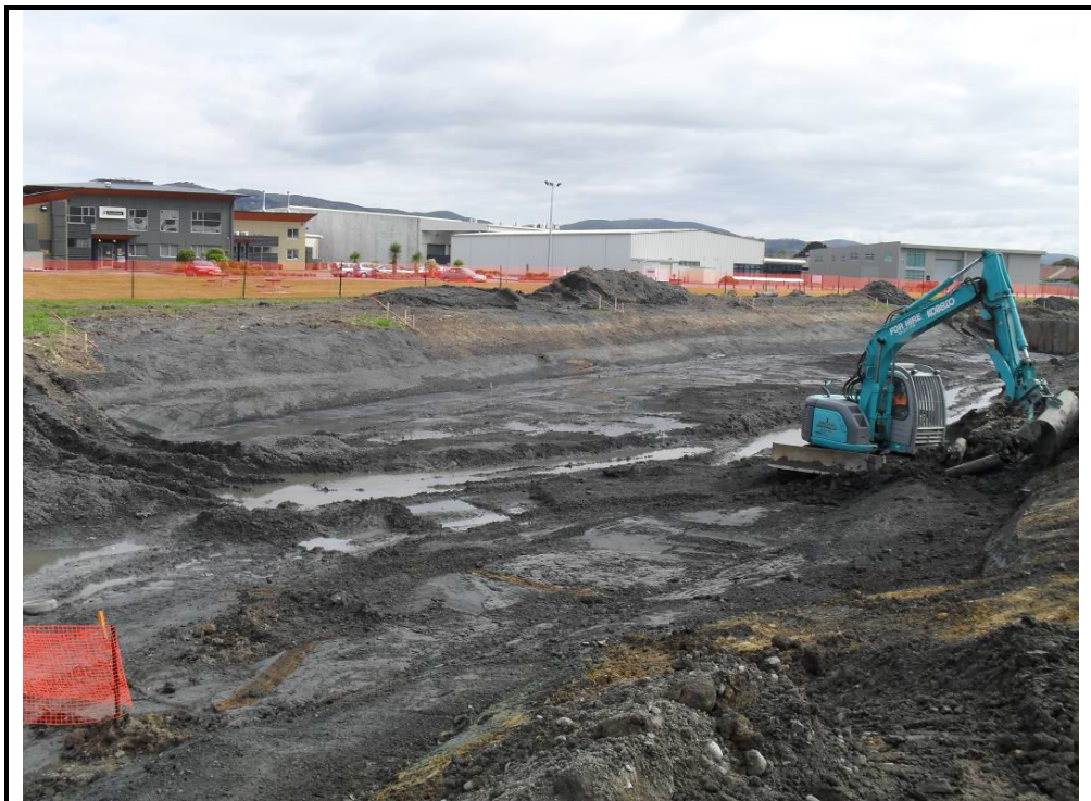
Photograph 4: The stream bed following the excavation of the contaminated material.
