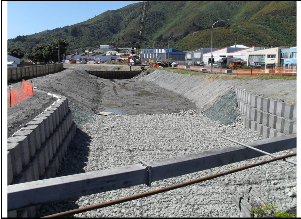
Photograph 7: Looking upstream towards coffer dam 4. Photograph taken from Hutt Park Bridge following excavation and installation of erosion and scour protection.
