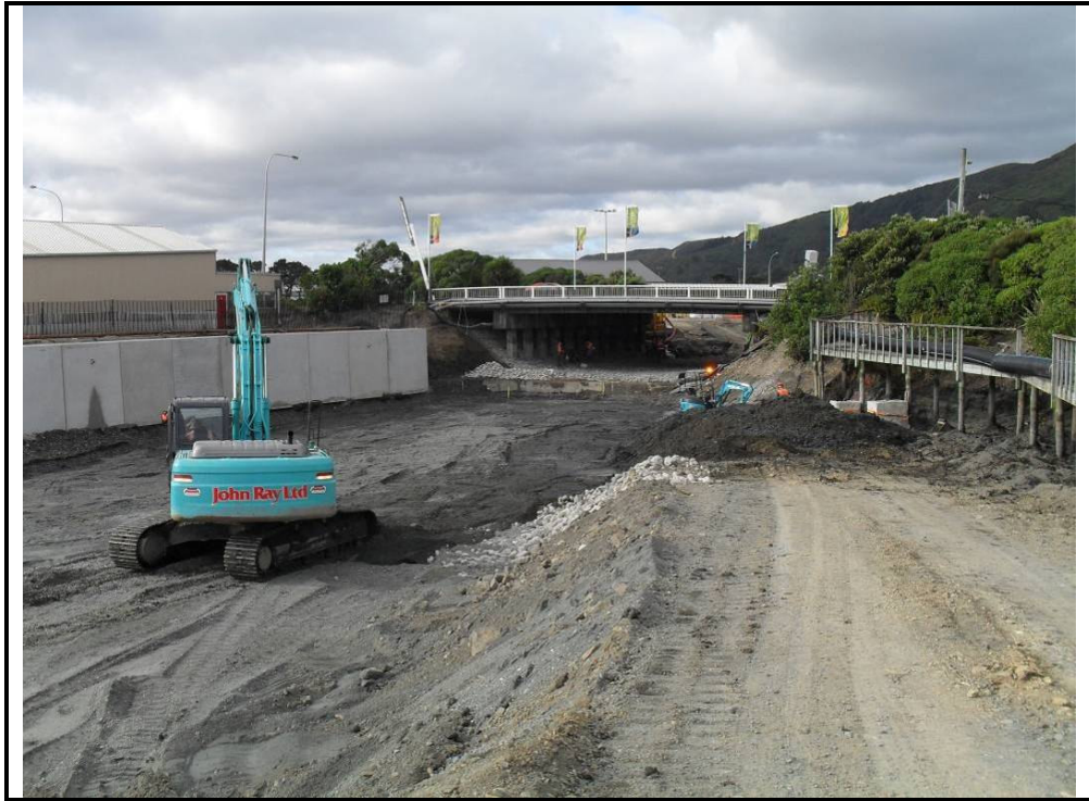
Photograph 7: View looking upstream towards Seaview Road Bridge of the salt marsh in Cell H following the removal of contaminated material.
