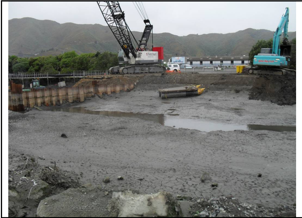
Photograph 1: Cell M immediately downstream of coffer dam 8 prior to the removal of contaminated material.
