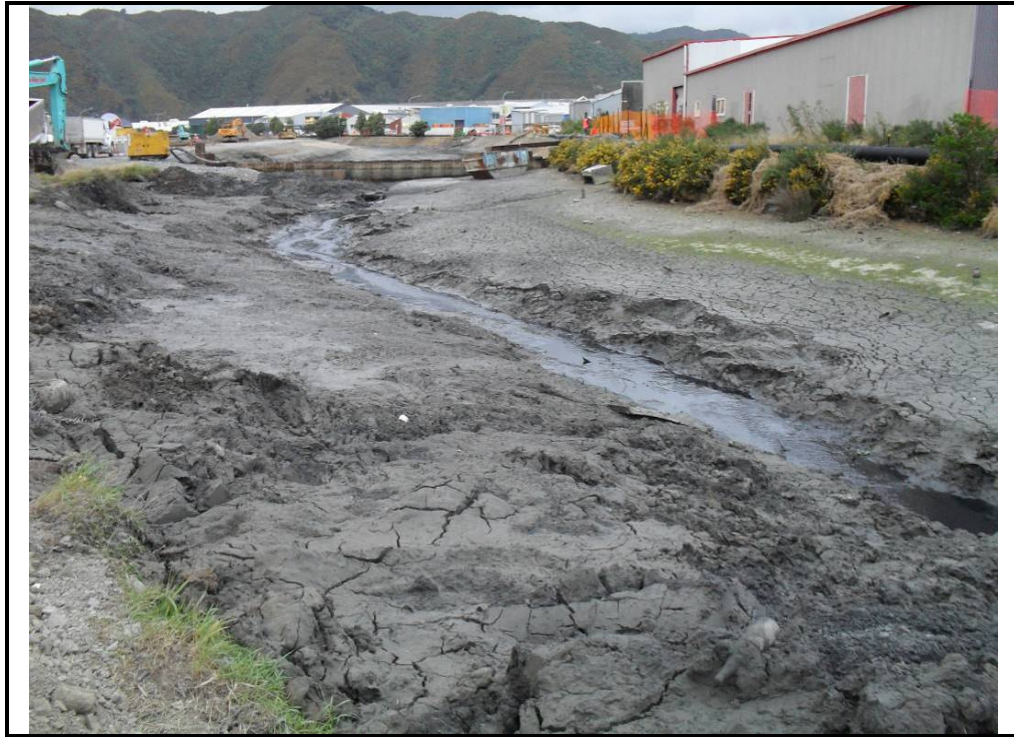
Photograph 1: Cell H looking upstream towards coffer dam 7, prior to the removal of contaminated material.
