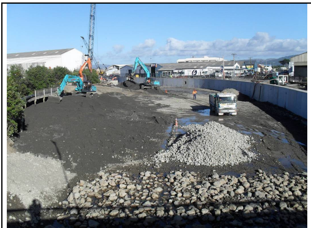
Photograph 8: View from Seaview Road Bridge looking downstream following the removal of contaminated material, and during the re-building of the salt marsh.
