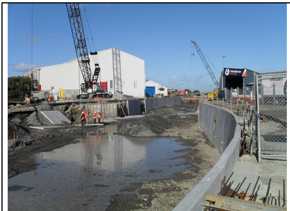
Photograph 4: Cell M (U-channel) looking downstream towards coffer dam 9 following the removal of contaminated material.
