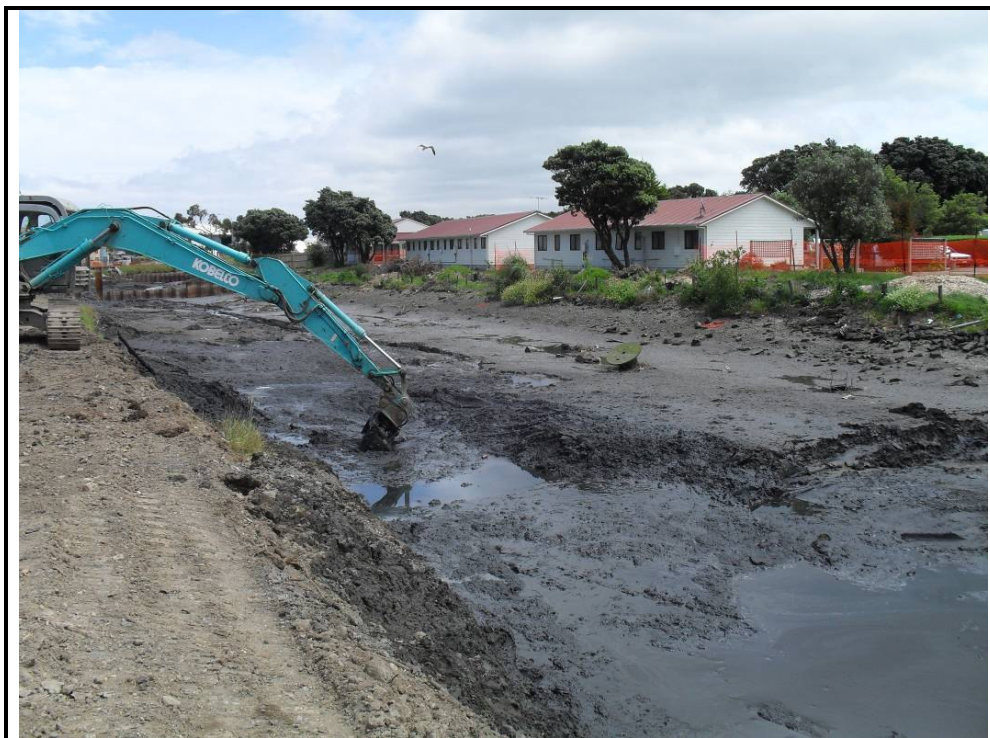
Photograph 1: Cell C during the early stages of excavation. Cofferdam 3 (in background) was removed during the works.
