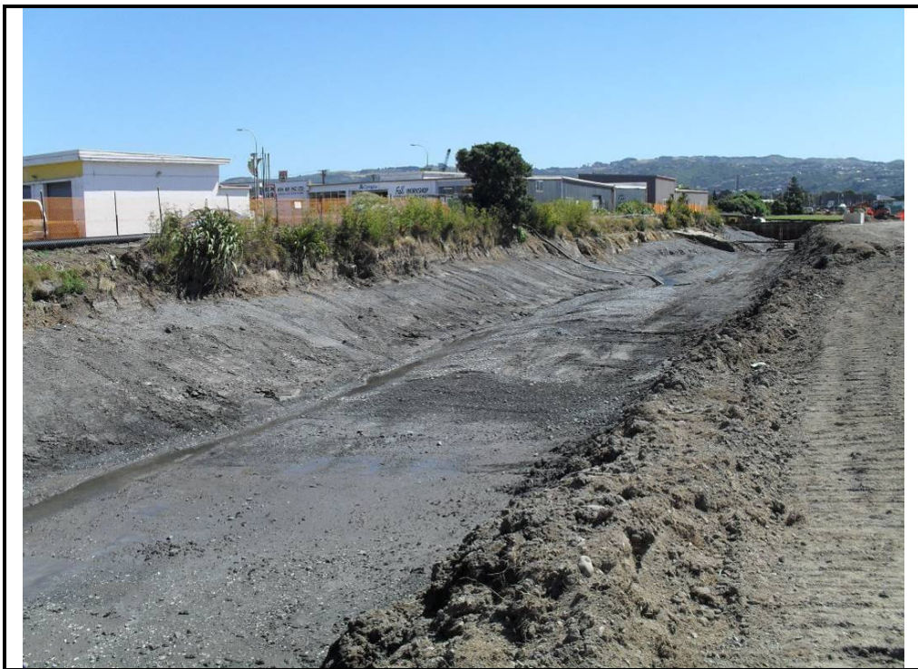
Photograph 4: View looking downstream towards coffer dam 7 following the removal of the contaminated material.
