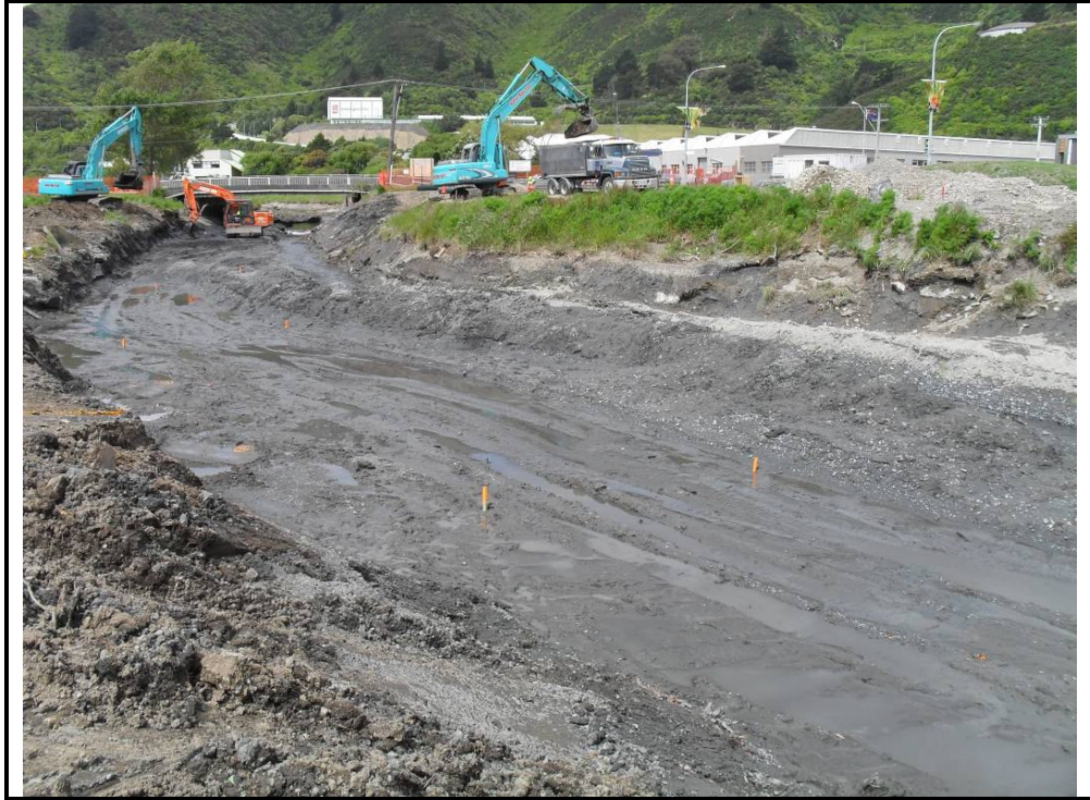
Photograph 3: Cell A, looking upstream during excavation. Orange pegs denote validation sample locations.
