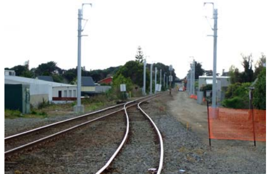
New traction poles heading north from paraparaumu
