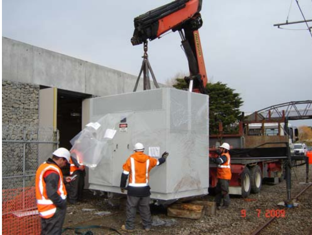
Electrical equipment being installed at Woburn
