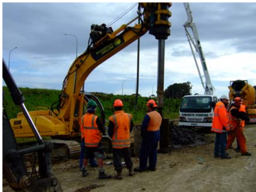
Drilling traction pole foundations near MacKays Crossing
