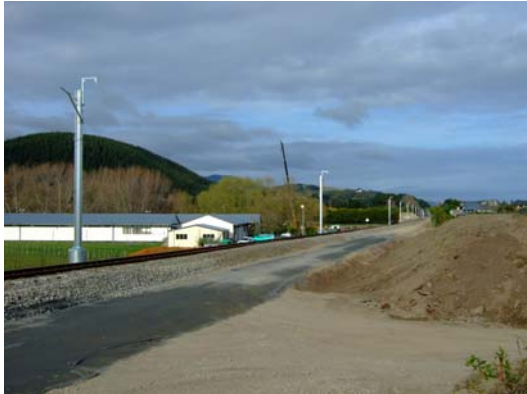
New traction poles near Lindale
