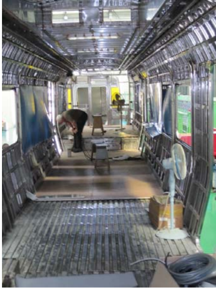
Matangi mock-up interior progress
