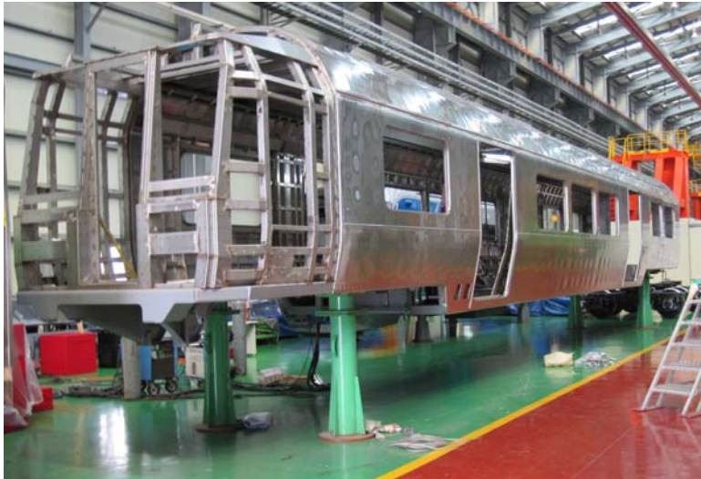
Matangi mock-up exterior progress
