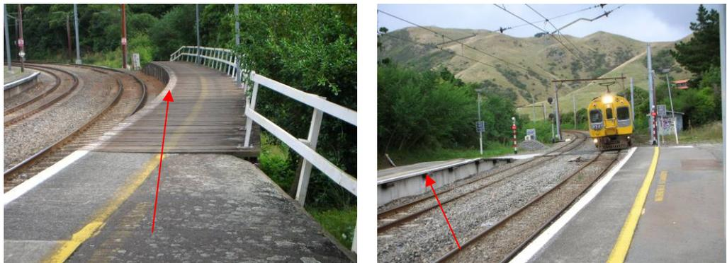
Figure 2. Muri Station – timber platform structure and temporary wooden reinforcement
