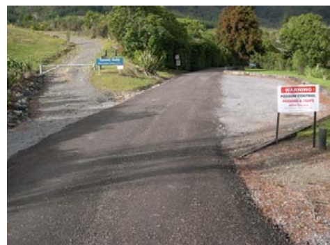
A section of Tunnel Gully access road, Pakuratahi Forest, surfaced with rotor millings
