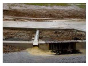
Silt discharge to stormwater at the Sunlink subdivision development.
