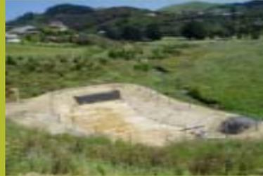
Sediment retention pond with flocculation, essential for sediment control at a subdivision site in Duck Creek, Porirua
