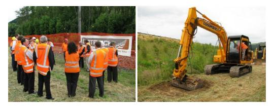
The drainage layer was installed at 'Preload Area 1' leading up to the Christmas break. Work continues at 'Preload Area 1' with the installation of many hundreds of vertical wick drains. These extract the water from the peat once the preload weight is applied. From January work will also commence at Preload Areas 2 and 3.
