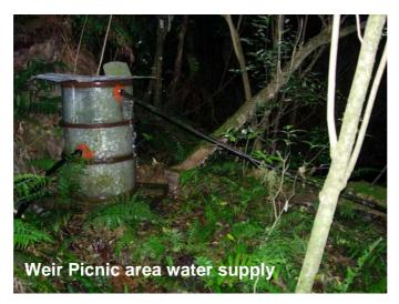
The Weir Picnic Area toilet water supply was fixed after it was damaged by vandals. This supply which is fed directly from Norbetts Creek is a great example of kiwi ingenuity and bush engineering and has provided a steady supply of water over many years. Siemens have repaired the power cabling under the Farm Creek ford that supplies the cell phone sites on the Hutt Water Collection Area access road.
