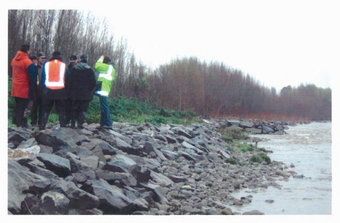
Linear Rock Lining with Debris Fences and Rock heads in background.
