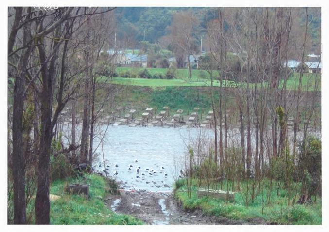
Newly erected Block Grid Patten and Willow pole structure.
