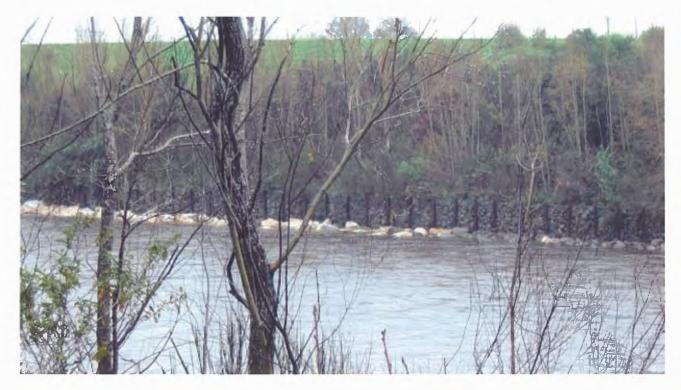
Longitudinal fence with rock placed along base.
