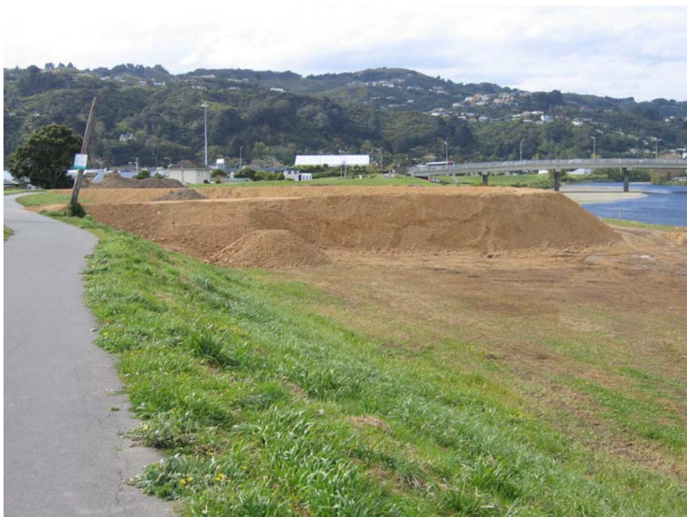
Showing the temporary Stopbank during an early stage of the works
