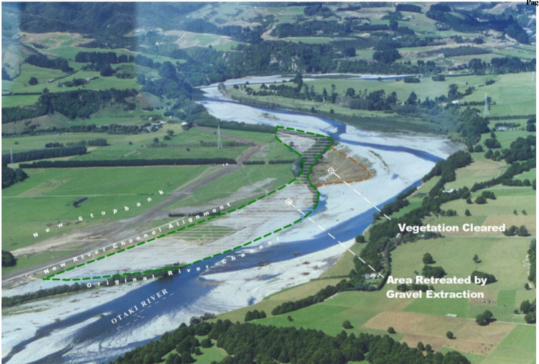
Photo of Upper Rahui Improvement Works
