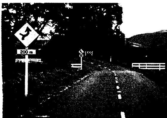
An unusual and potentially confusing array of signs approaching a moderate curve.
