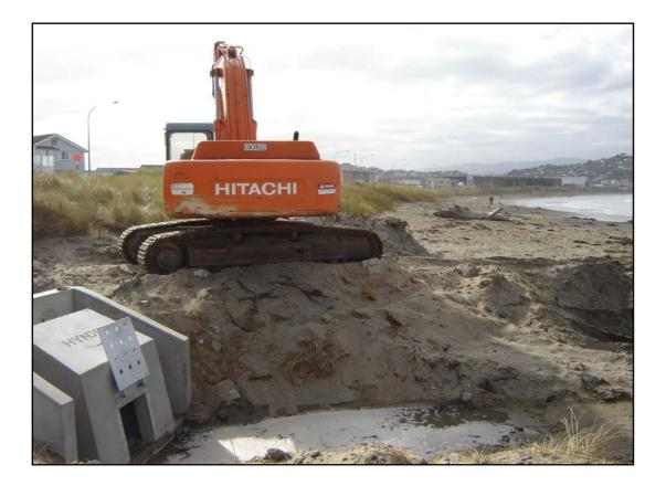
Figure 11: Stormwater pipe upgrade construction underway in April 2009. Note the stormwater outlet is several metres landward of the vegetated toe of the foredune visible in the background.
