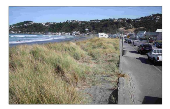
Figure 10: Area D showing seawall, windblown sand on the footpath and the marram grass dominated foredune.
