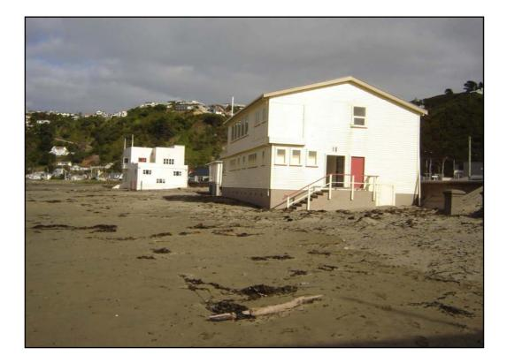
Figure 13: AREA 5 showing buildings located seaward of the seawall that are clearly within the active foredune zone. The relatively flat beach is highly vulnerable to storm waves reaching the buildings and seawall.
