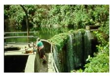
The dam operated until the Kaitoke Scheme commenced supply in 1954. The dam continues to retain a lake, however the volume of the dam has decreased over the years because of silting. In 1988 the dam was drained and silt was measured to 6.3 metres below the spillway. Eels and some brook trout now inhabit the lake.
