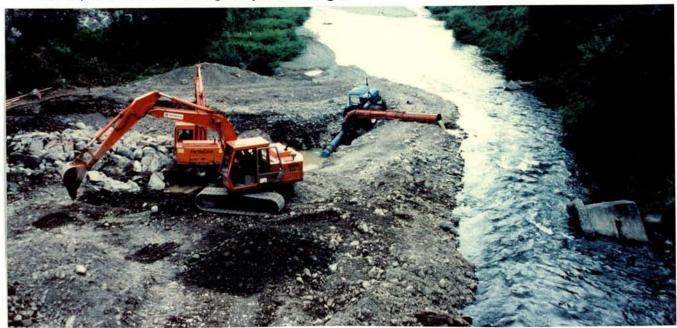
Figure 7. Ministry of Works construction of the Waikanae weir to control bed levels downstream of the state highway bridge. The rock weir replaced a concrete block weir that had been constructed and maintained by the catchment boards.
