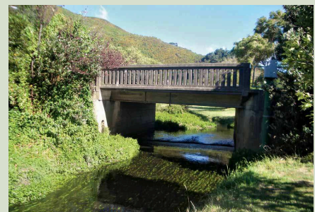
White Lines East Road Bridge
