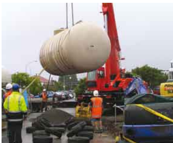
We have increased our diesel reserve at Waterloo following the installation of a new storage tank.
