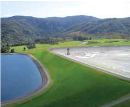
The northern storage lake at Te Marua was empty until late November, to carry out repairs.
