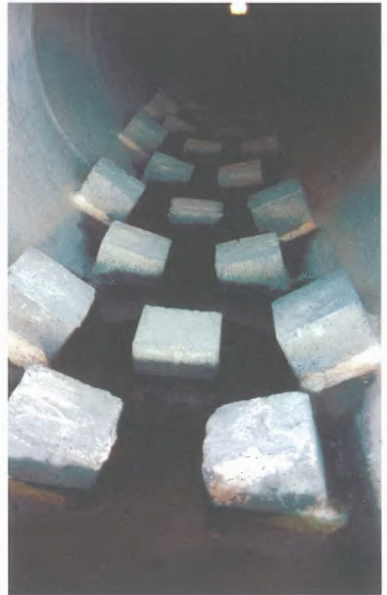
Concrete blocks attached to a culvert floor are fish-friendly
