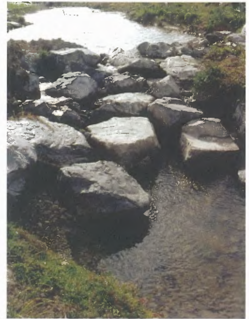
A rock ramp on a small stream is more fish-friendly than a vertical concrete weir
