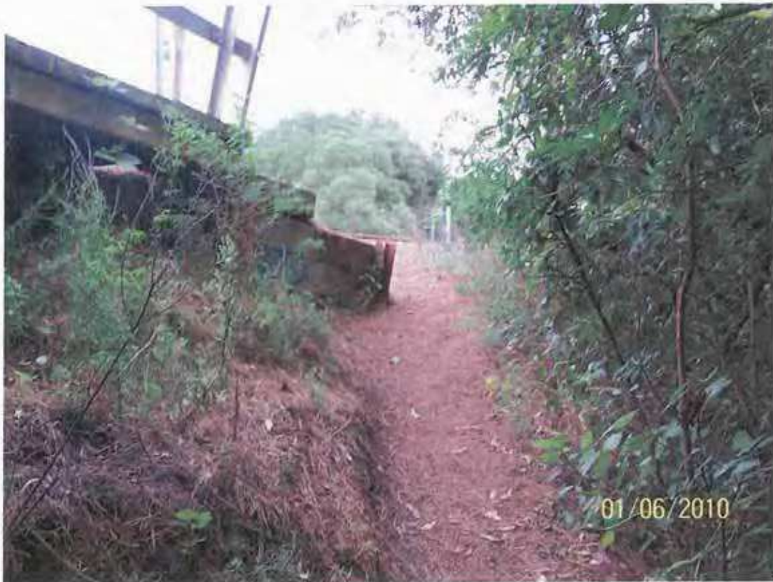
Photo 11 – Up platform southern end – illegal access point
