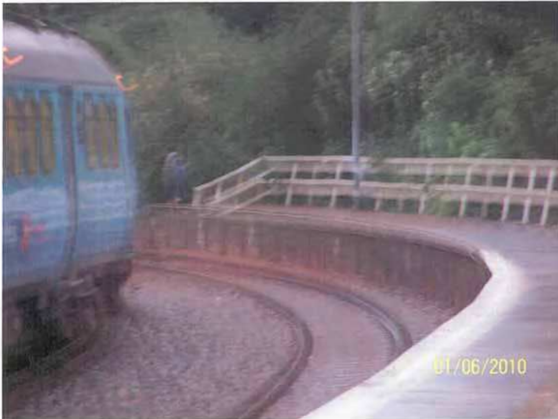
Photo 19 – Up platform southern end – illegal access point in use
