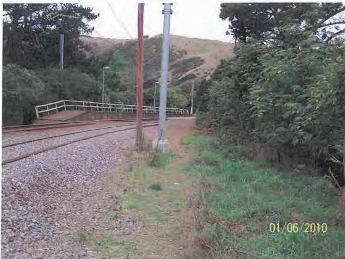
Photo 17 – Down platform southern end – illegal access point
