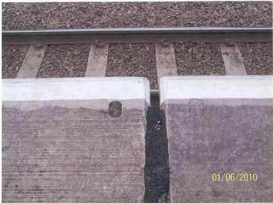
Photo 6 – Up platform platform edge defect
