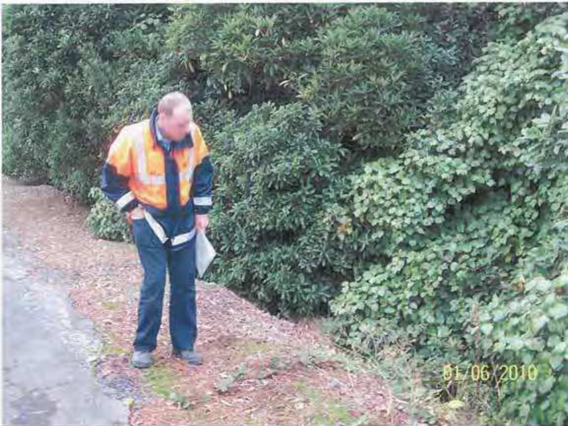
Photo 16 – Down platform – unprotected bak of platform
