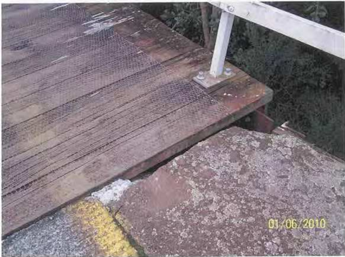
Photo 8 – Up platform timber to concrete platform transition
