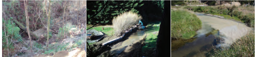
Figure 2: Photographs relating to enforcement actions taken during 2010/11. From left: deposition of fill material in a watercourse, placement of a concrete block erosion protection wall, discharge of sediment to a watercourse.
