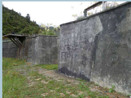
Repaired lower dam
