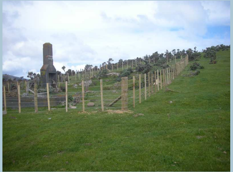
New fencing around Baring Head structures
