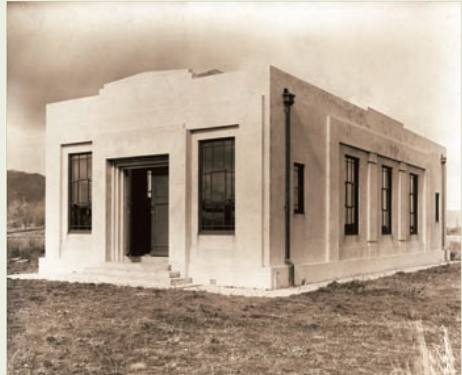
With a hint of stripped classical and deco simplicity, the architectural Gear Island pumping station was built in 1935. It is still in use, albeit with the windows filled in.
