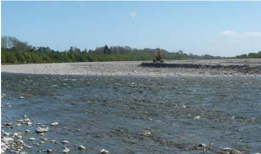
Figure 2.5: Gravel extraction and channel control works at Chrystalls Bend
