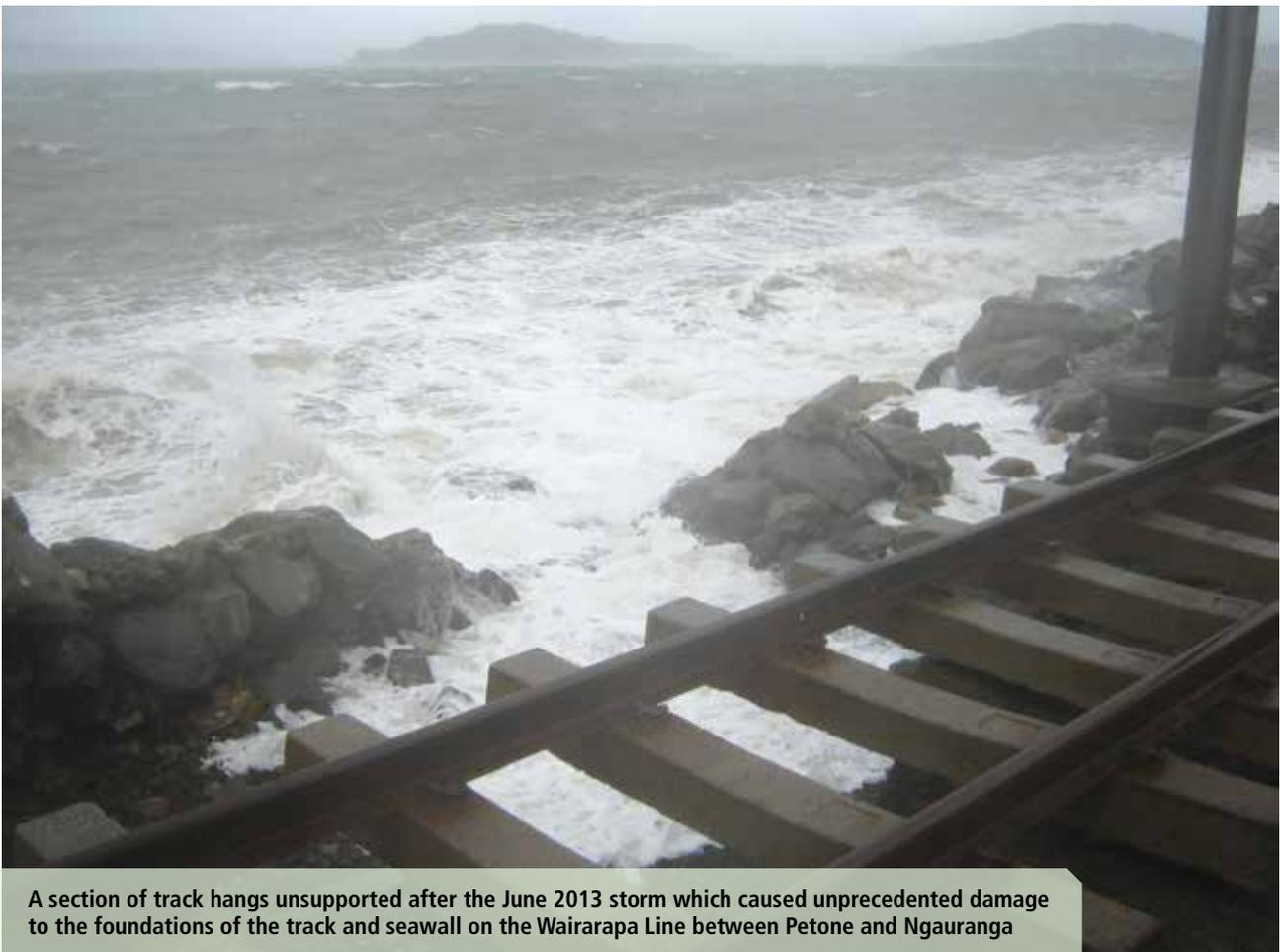
A section of track hangs unsupported after the June 2013 storm which caused unprecedented damage to the foundations of the track and seawall on the Wairarapa Line between Petone and Ngauranga
