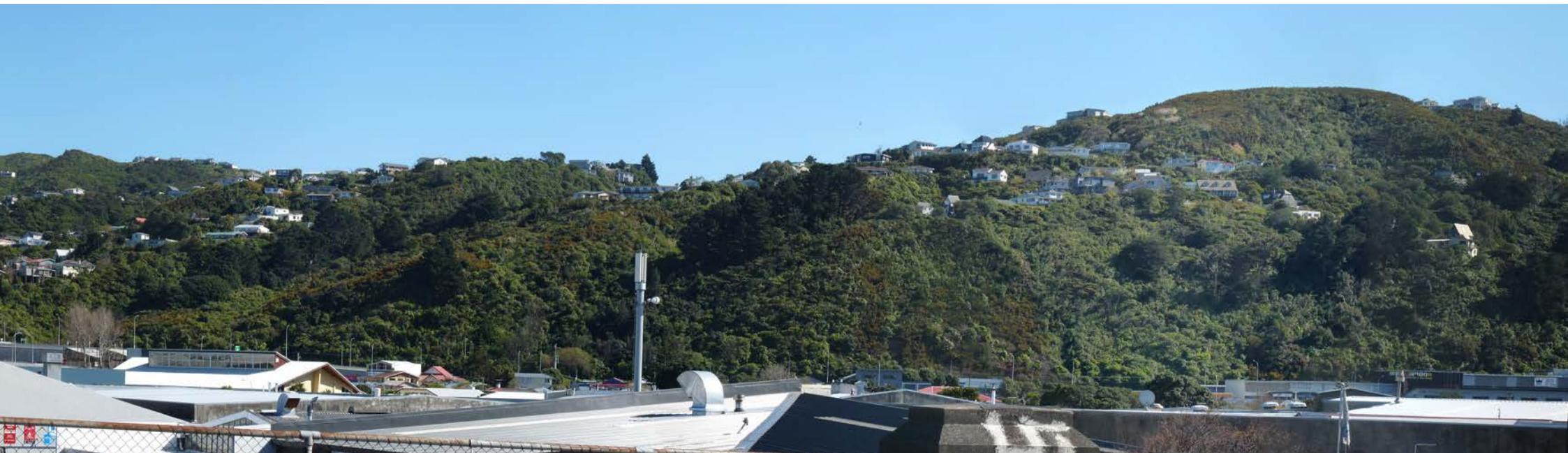
The Western Escarpment is peppered with residential dwellings that are nestled into the hill slopes.
