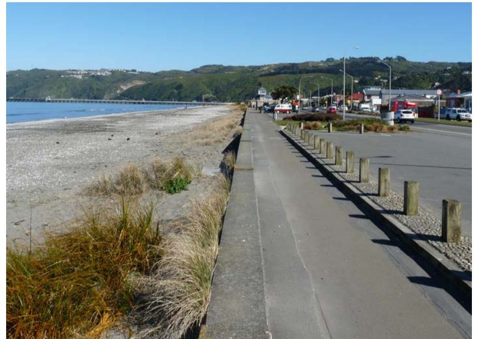
The Petone foreshore forms the south-western boundary of the character area.
